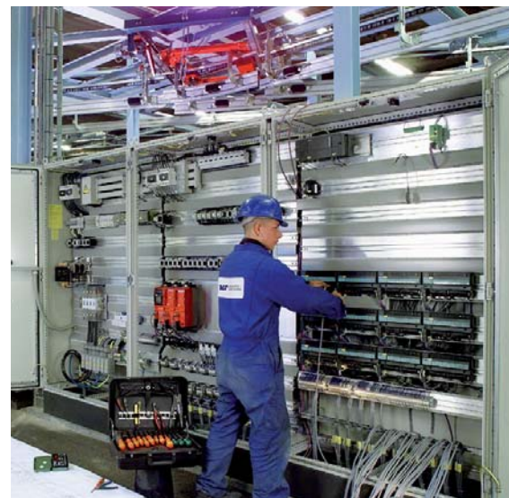
Switch cabinet manufacturing
