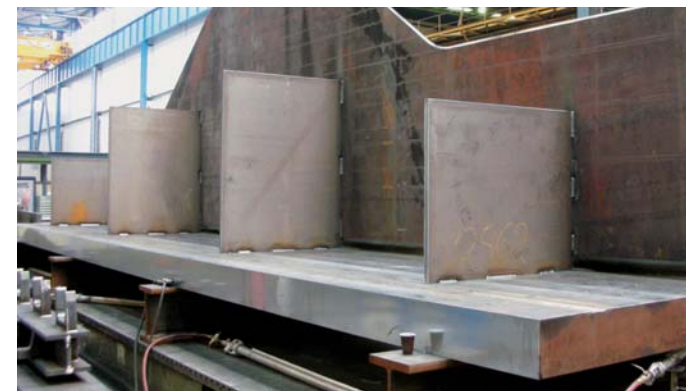
Welded construction of an upper beam
